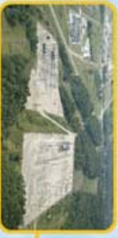
Don Marquis Substation
