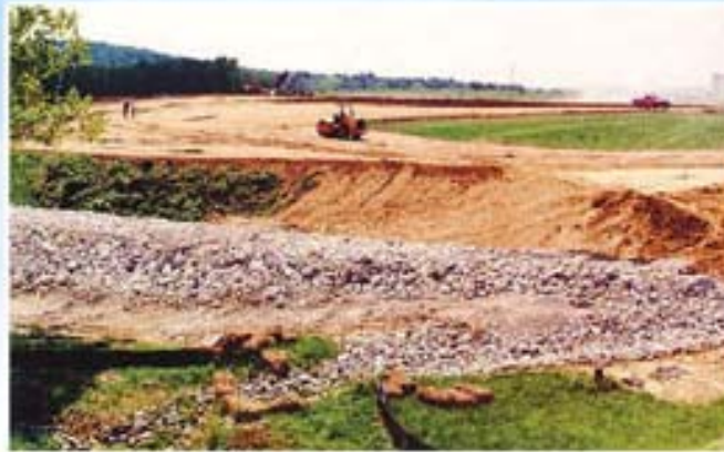
X-749B (Peter Kiewit) Landfill Closed and Capped - 1998
