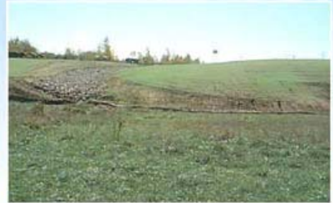
X-734 Construction Spoils Landfill Closed and Capped - 2000
