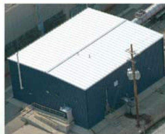
Pictured above is an aerial view of the X-627 Groundwater Treatment Facility. Below: Several of the 3,000 hybrid poplar trees planted as part of the phytoremediation project on the southern edge of the plant site.
